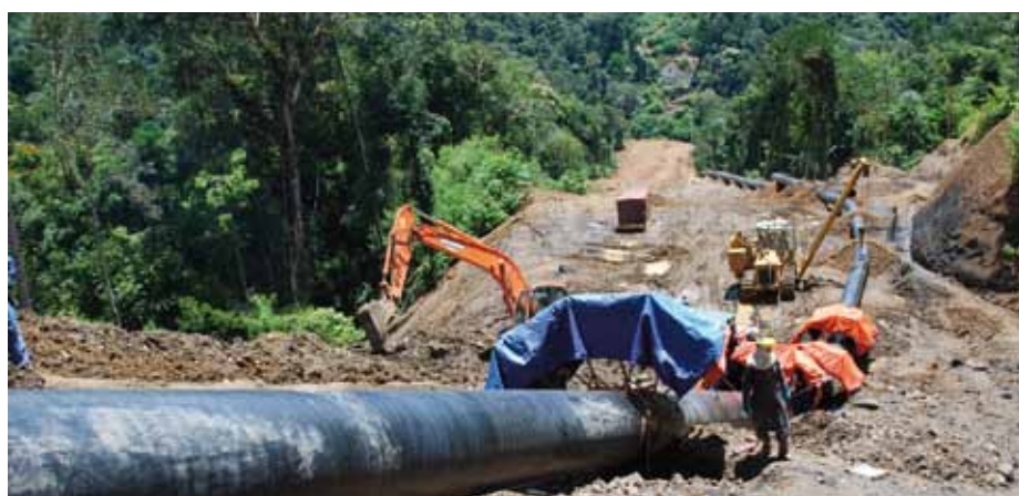
Automatic welding of the SSGP project.
