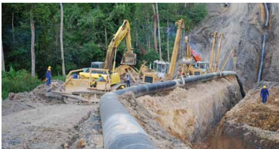
Preparing to lower-in the SSGP.
