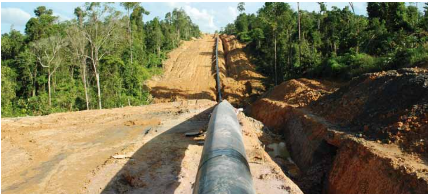
The welded pipeline alongside the trench.
